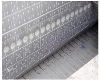
thick, and on a liner with 15mm of wear material, the potential available life could be up to five years. In the image below, the casting markings can clearly be seen – indicating that in some cases, the only material that had worn off the liners was the paint.
